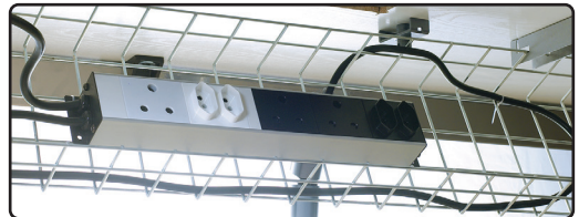
Custom brackets allow the cable tray to be un-clipped and swung down.
