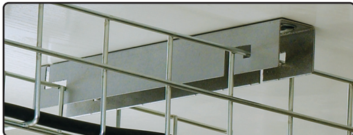
Custom brackets allow the cable tray to be un-clipped and swung down.
